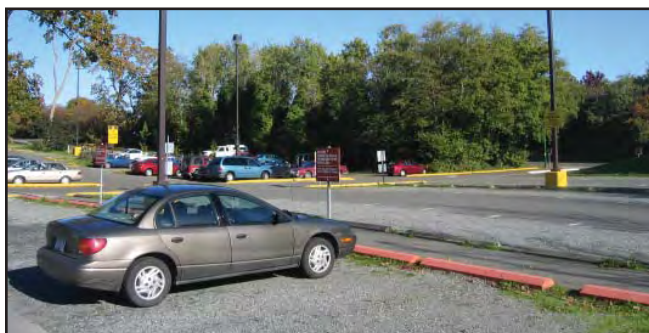
Image of typical gravel parking stall and paved drive aisles
